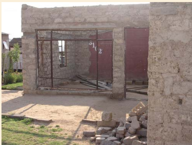
Building bit by bit to add a room on to an RDP house in Diepsloot, South Africa
